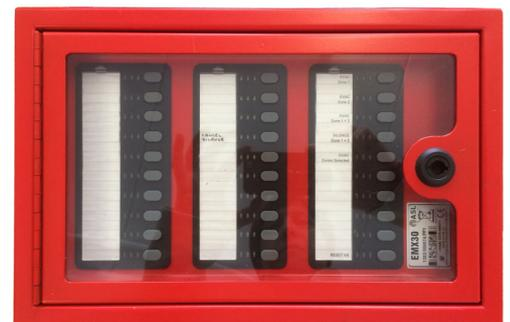
Top, bottom and rear cable entry points are provided by means of 'knock-outs' in the enclosure, while the field connections are provided by means of a set of terminals on the inside rear panel of the back box. The EMS10, EMS20 and EMS50 are compatible with the whole range of ASL Voice Alarm and Public Address systems, and are designed to comply with EN54-16, ISO 7240-16 and BS5839-8.
